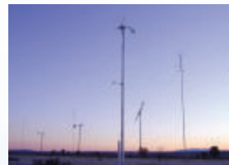
CIEMAT-CEDER test facility (Sora), Spain (in collaboration with )
