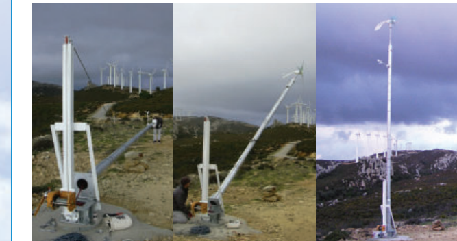
Lying down Lifting with the specialized winch Final position
